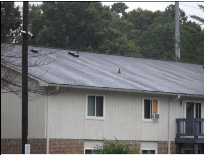
39. Pitched roof with shingles are provided.
