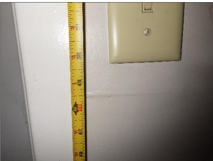
65. Designated accessible unit light switch; note height exceeds 48" AFF.
