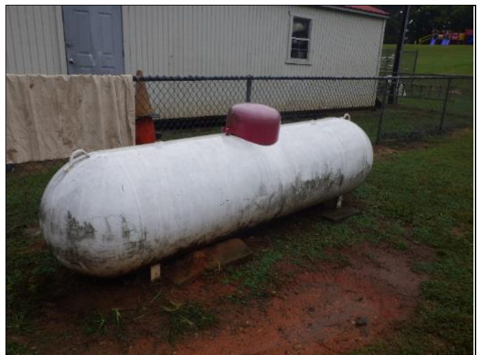
60. Propane tank for laundry room equipment.
