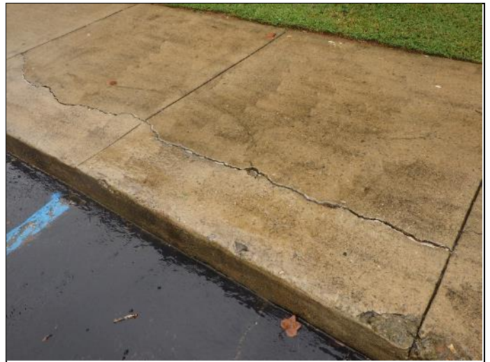
10. Cracked sidewalk by G building and trip hazard.
