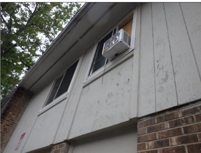
29. T1-11 wood siding is used on each building.
