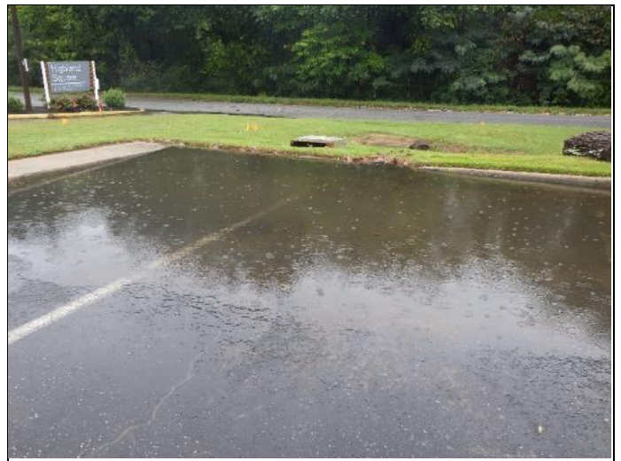
4. Ponding of water near F building.
