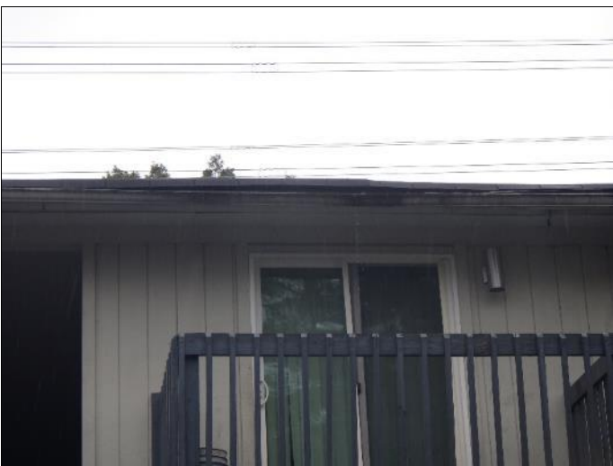
41. Roof drainage; note gutters in poor condition and need to be replaced on each building.
