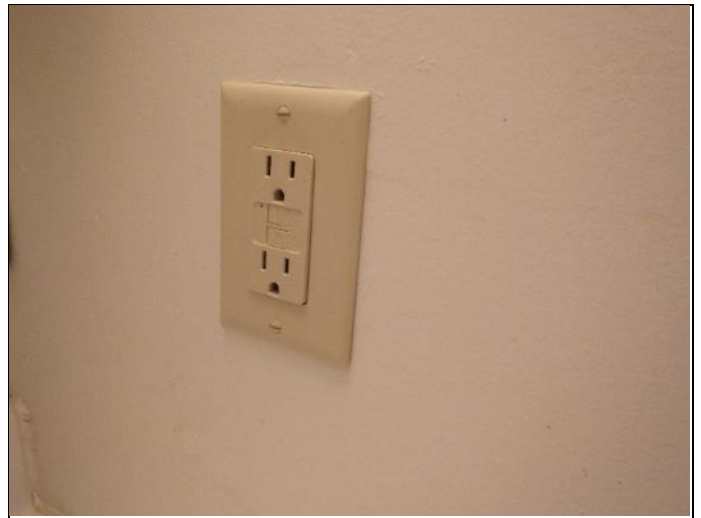
52. GFCI outlets are provided in each unit.
