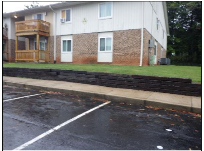
16. Crosstie retaining walls are provided.
