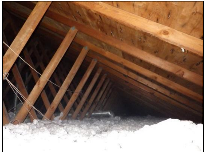
22. Wood framing and sheathing is used.
