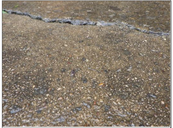
8. Trip hazards found at most building walkways.
