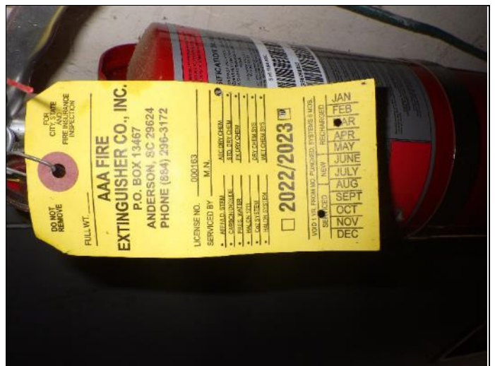
54. Extinguisher with expired tags; in common areas only.
