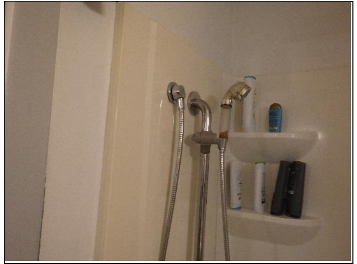
68. Designated accessible unit; wand-type shower head provided.
