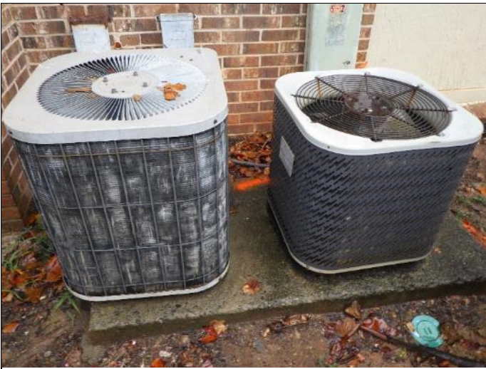
45. Split system condenser units.
