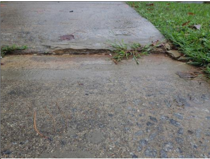
9. Typical displaced sidewalks throughout the site.
