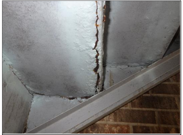
32. Cracked steel treads need repairing.
