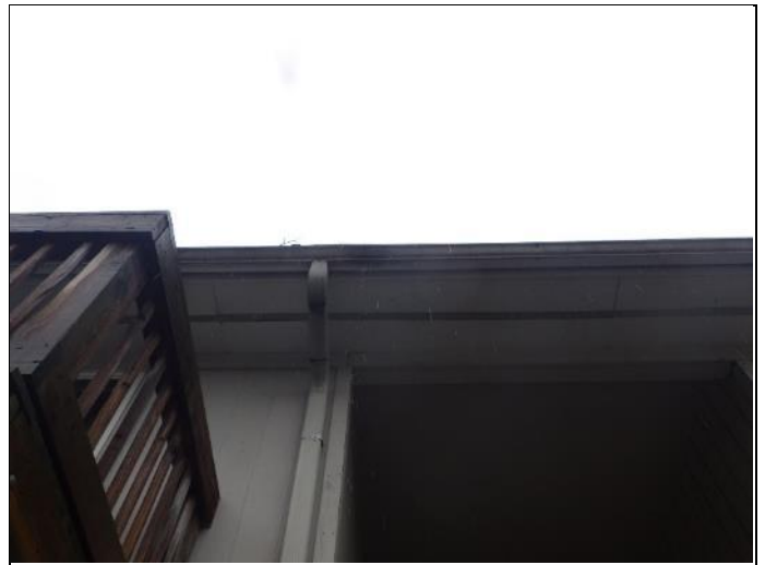
40. Roof drainage; note gutters in poor condition and need to be replaced on each building.
