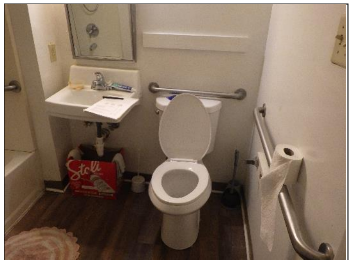
66. Designated accessible unit bathroom; note missing ptrap cover.
