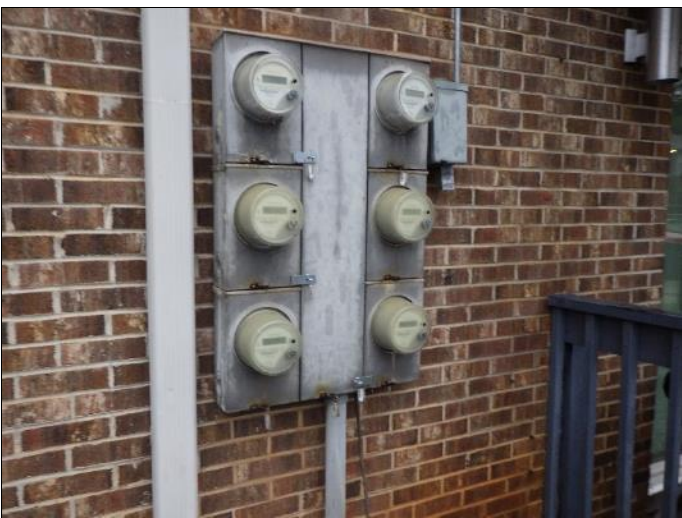
47. Individual electrical meter bank.
