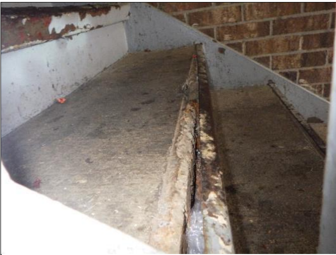
33. Corroding stair system needs repairs.
