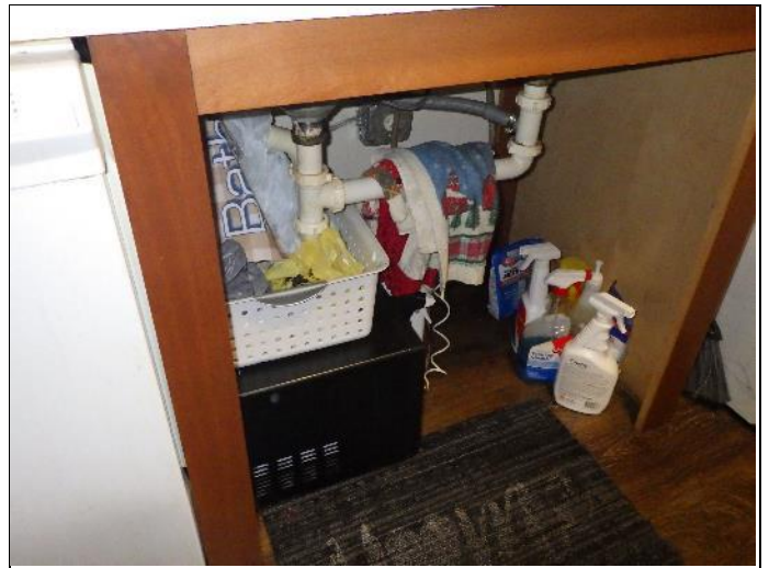
64. Designated accessible unit kitchen; note lack of pipe cover.
