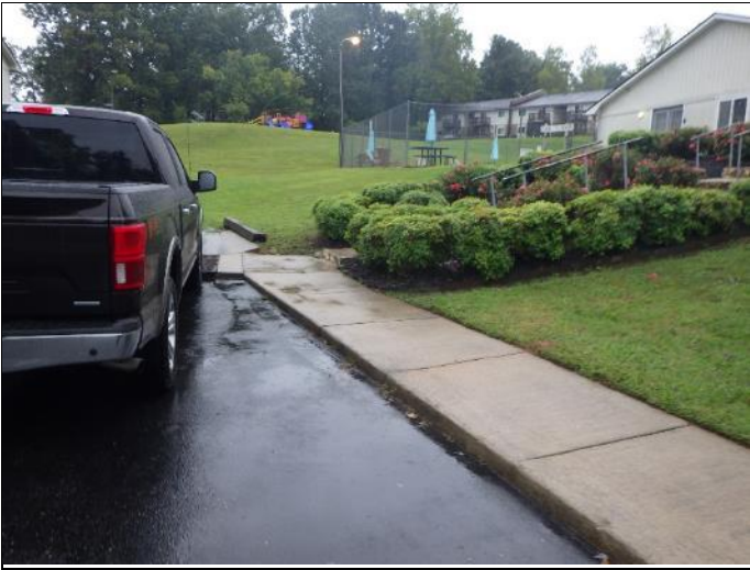
13. A curb cut is needed for accessible route to the leasing office.
