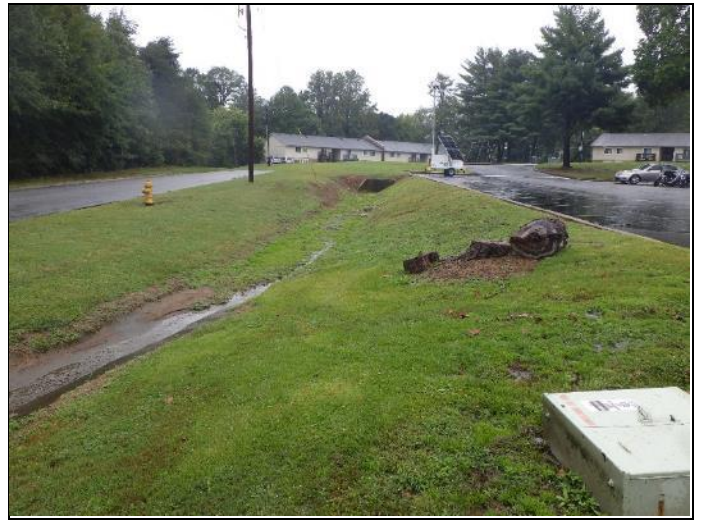
2. Storm drainage ditch to municipal system.
