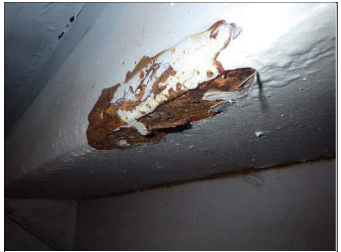
34. Corroding stairs need repairs.
